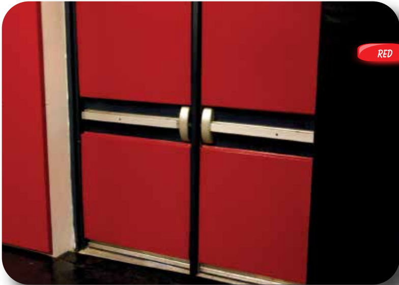
CUSTOM PADDING Custom pads designed for this door allow the emergency bars to still function properly.
