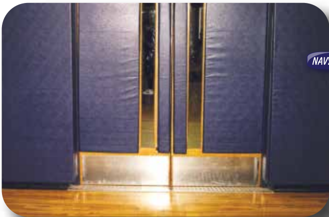
CUSTOM PADDING Custom pads for this door were added without blocking the windows and leaving the bottom kick plate unpadded.
