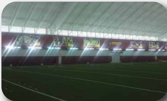
Wall padding for the new indoor practice facility in Ames, Iowa, for Iowa State University.
