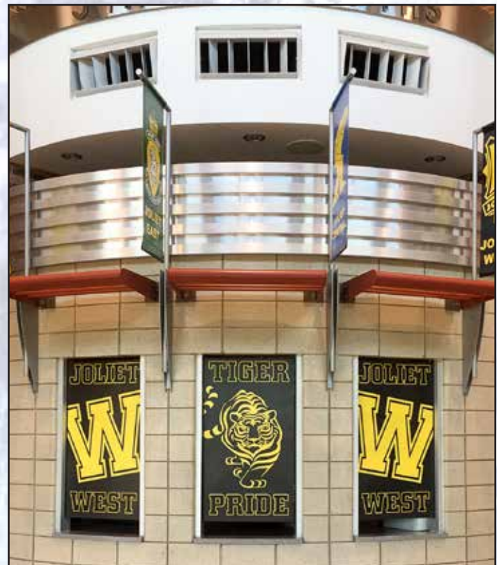
JOLIET HIGH SCHOOL WINDOW VINYL BLOCKING UNUSED WINDOWS
